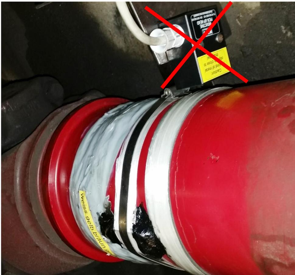
Wrong installation, head position is 90° wrong to the coil and will not work!
